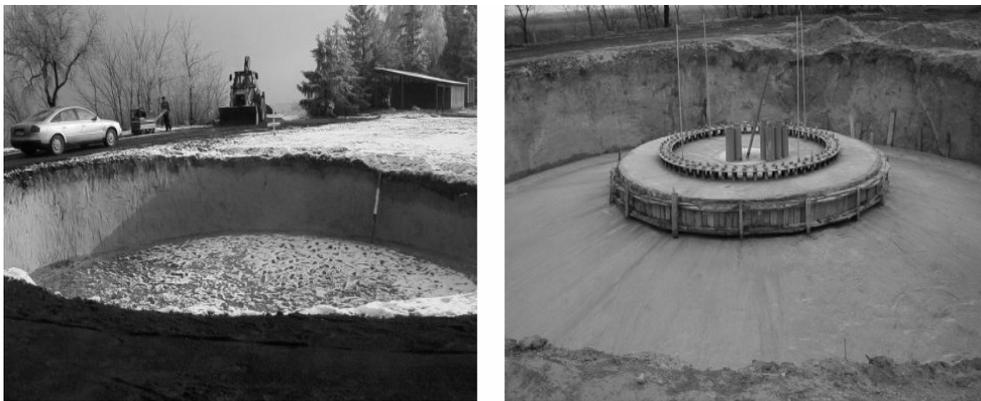
*Fig. 1* Phases of laying the foundations for the wind turbine at Kulcs
